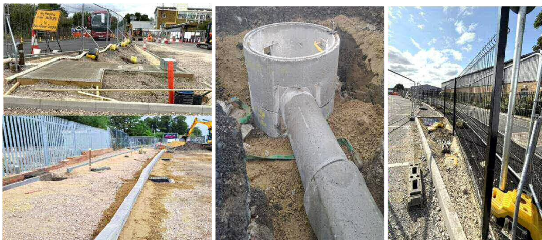
Phase 3 progress with kerbing, fencing, foundation construction and drainage works
