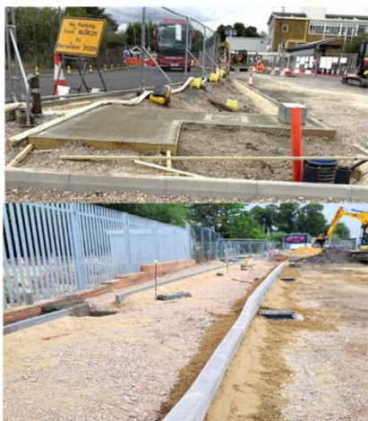
Phase 3 progress with kerbing, fencing, foundation construction and drainage works
